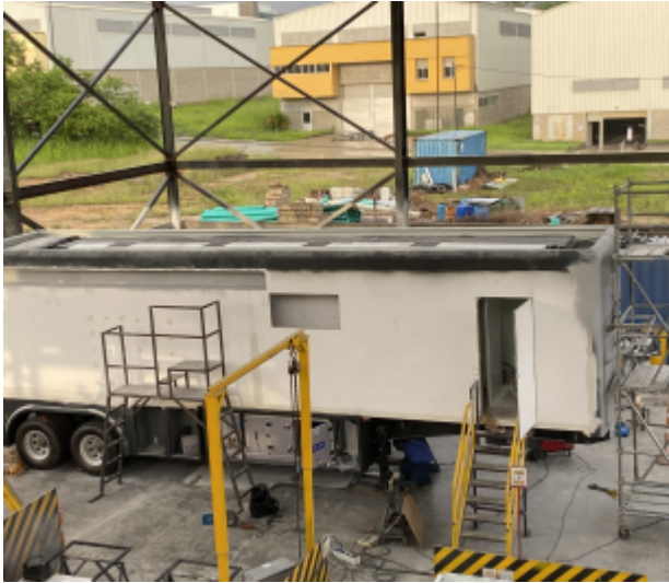
Aerial view of the laboratory body during fabrication at NINOX's Cali facility, November 2020. The aluminum sandwich structure with high-density thermal insulation core is visible in the assembly stage.
