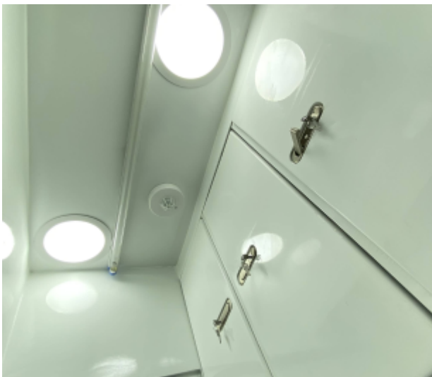
Interior module view: flush-mounted circular LED panels, germicidal UV tube, and industrial lever-lock storage cabinets. The clean geometry eliminates surfaces that are difficult to decontaminate.
